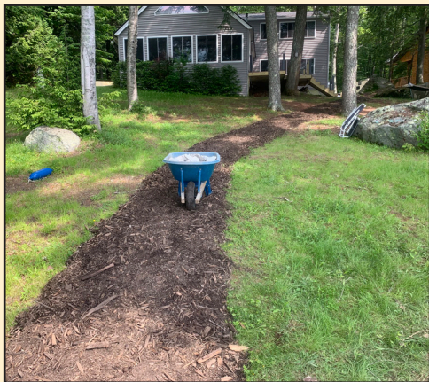
Erosion Control Mulch
