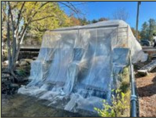
The nylon dome allowed a tented and dry environment in which to work.
