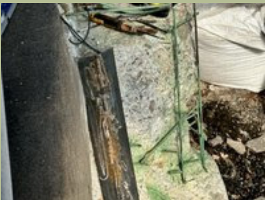
Note the new north abutment welded rebar awaiting the concrete truck.
