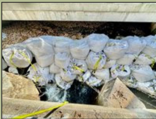
The cofferdam was constructed of fifty 2,500-lb. sand bags.
