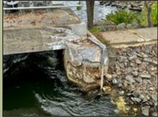
Note the deterioration of the north abutment concrete.
