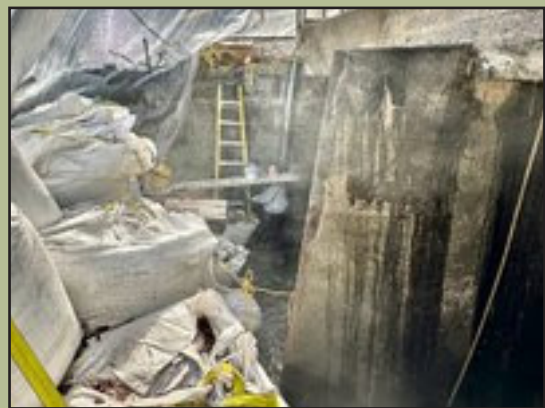
The cofferdam was constructed of fifty 2,500-lb. sand bags.
