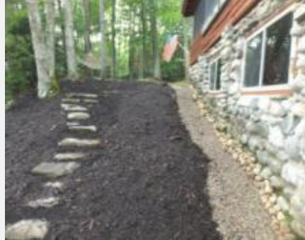
Dripline trench & erosion control mulch (Photo: AWWA)
