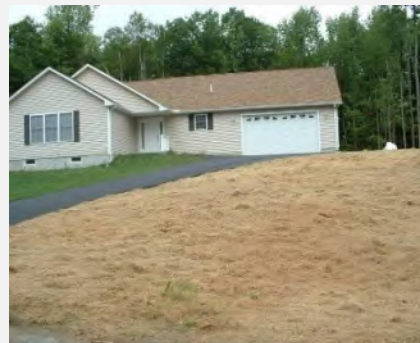
Install permanent BMPs once construction is complete including seed/ haying bare soil and installing vegetation on the shoreline (Photo: Maine DEP)
