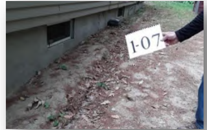
Roof dripline erosion at a residential site in Sector 1.
