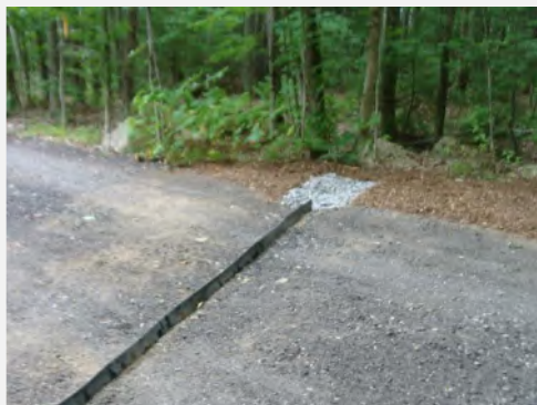
Reshape gravel roads, add new surface material, and install runoff diverters
