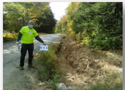
A roadside ditch in Sector 9 requires vegetation and re-shaping to prevent sediment from flowing into the lake.
