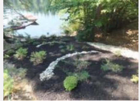
Erosion control mulch & vegetative planting
