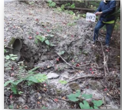
Sheet erosion and an unstable culvert in Sector 10.
