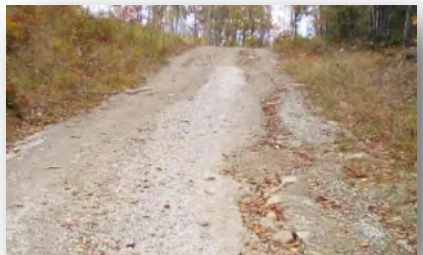
Gully erosion on Vienna Mountain Road in Sector 4.
