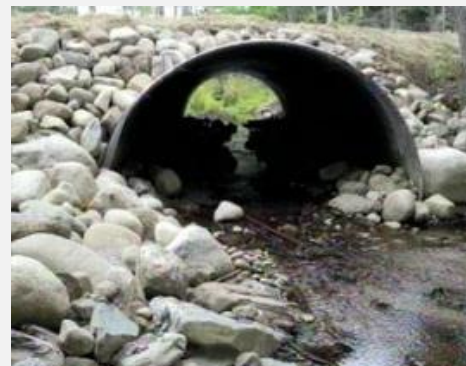
Replace undersized and perched culverts, remove clogs, armor inlets/outlets and install plunge pools
