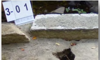
A sink hole on the Watson Pond Road crossing in Sector 3.
