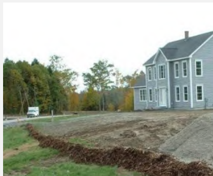
Install temporary BMPs such as an erosion control mulch berm prior to beginning construction
