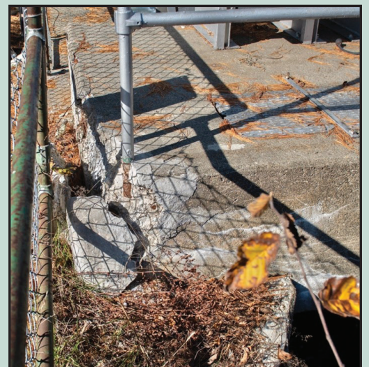
The concrete deterioration is throughout.
