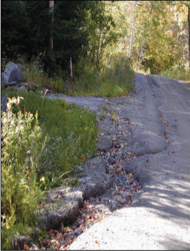
Figure 13. A diversion of some type and a ditch to carry water away from the road are needed to stop the erosion that has already occurred in the image taken during the road problem survey on 19-Sep-06.
