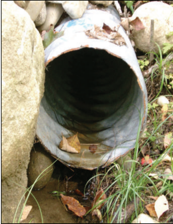
Figures 11 and 12. The picture on the left is a representation of a good culvert with proper drainage and depository pool taken during the road problem survey on 19-Sep-06. The picture on the right is a representation of a poorly maintained culvert as it is filled with debris, has no room for runoff, and no collection pool observed during the road problem survey on 19-Sep-06.
