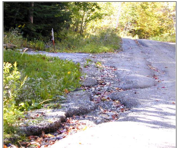
Example of a camp road in the Long Pond south direct watershed with poor crowning. (Photo: CEAT)
