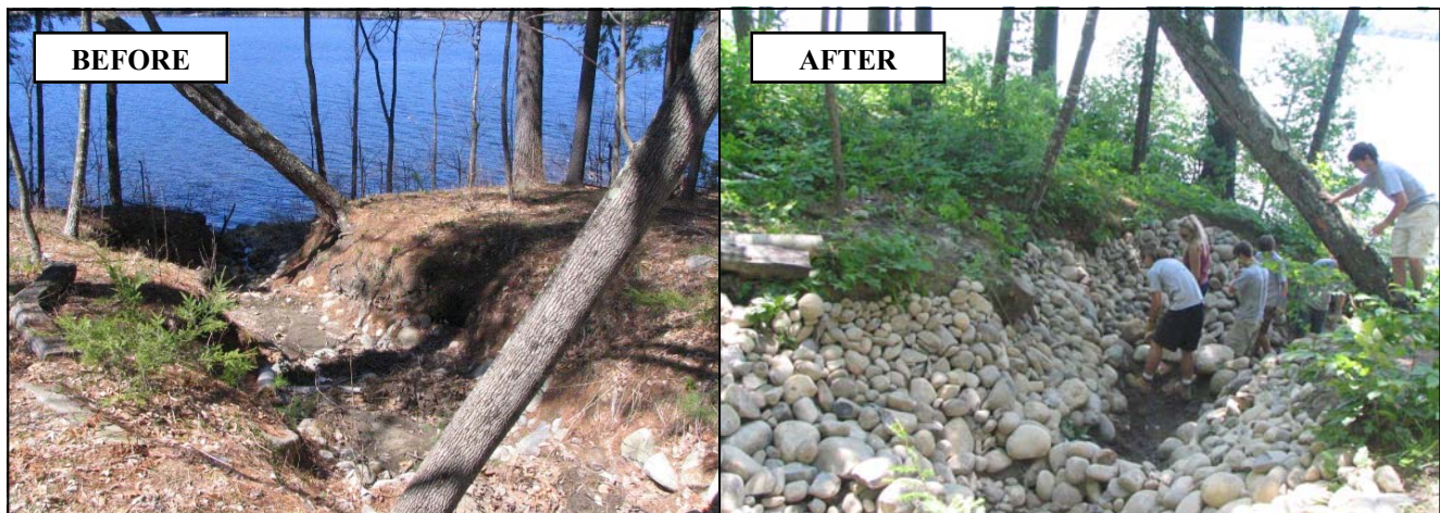
The BRCA Conservation Corps has actively installed BMPs in the Long Pond Watershed since 1996. A recent BRCA project (above) involved armoring a badly eroded ditch carrying large amounts of sediment from Rt. 27 into Long Pond (Photo: Jason Bulay).
