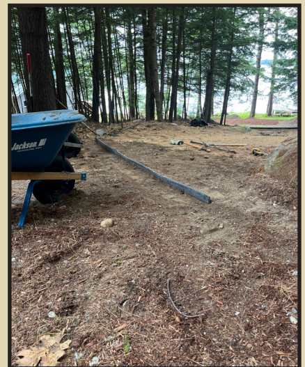
Stormwater run-off controls are in place.
