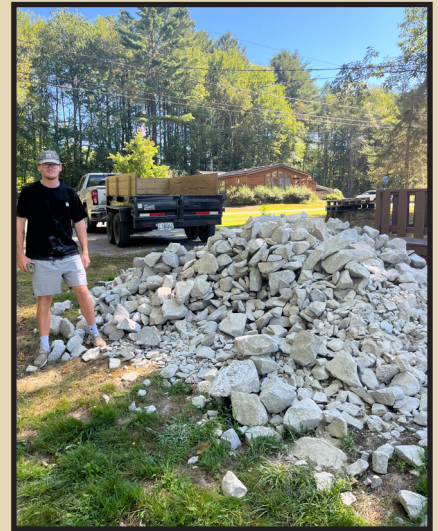
Rip rap halts shoreline erosion.
