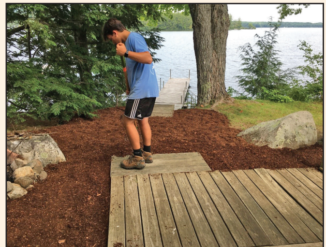
Installing erosion control mulch on path to the lake
